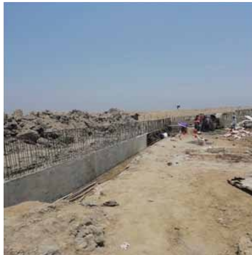
Fig: Construction of Retaining Walls for Approach Road
