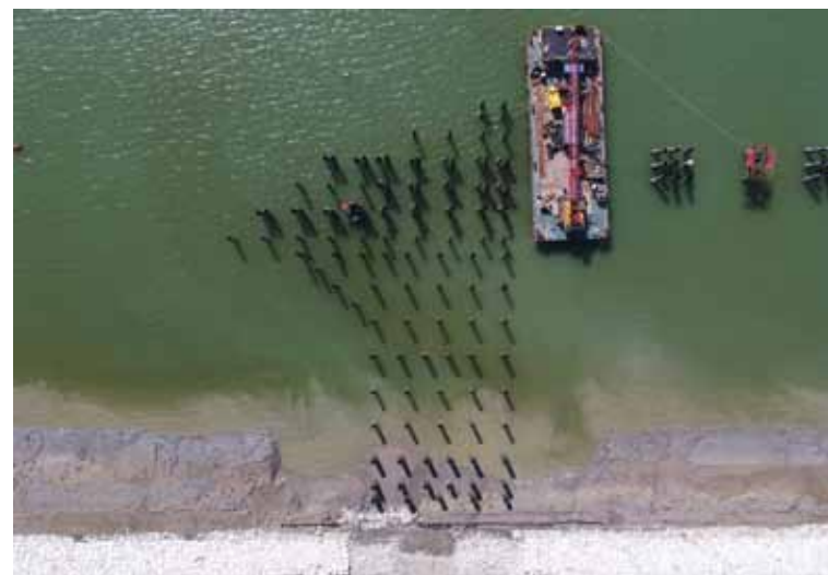
Fig: Piling works of Coal Unloading Jetty
