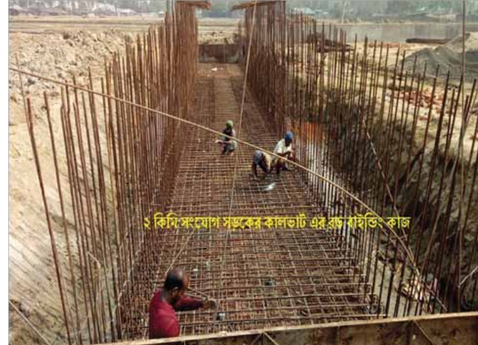
Fig: Construction of Culvert for Approach Road
